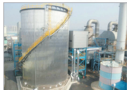
Pressure Maintaining System: Paju Combined Heat & Power Plant Construction Project Project Owner : Korea District Heating Corporation Contractor : Daewoo Engineering & Construction Pressure Maintaining System: 90mL x 2 units
