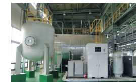
Pressure Maintaining System: Paju Combined Heat & Power Plant Construction Project Project Owner : Korea District Heating Corporation Contractor : Daewoo Engineering & Construction Pressure Maintaining System: 90mL x 2 units
