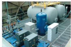
Seongnam Resource Recovery Facility Reconstruction Project Project Owner : Korea District Heating Corporation Contractor : Kenertec Pressure Maintaining System: 1.5mL x 2 units
