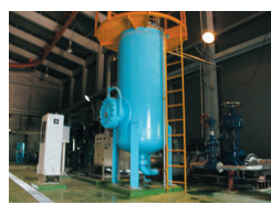
Project Name : Taebaek Seohak Leisure Complex Snow Making Water 570kw x 630mAq x 6pumps
