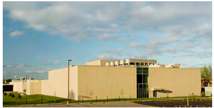
Applied Development Center
