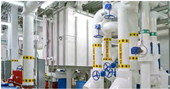
Applied Development Center
